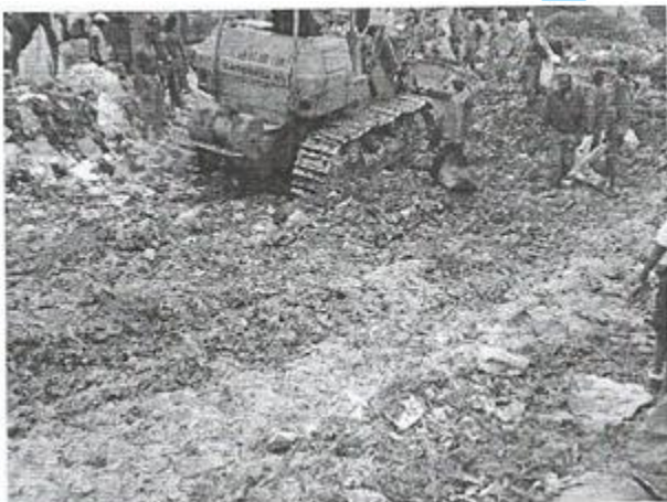
Figure 7: Bulldozer compacting after the waste picker has finish sorting
